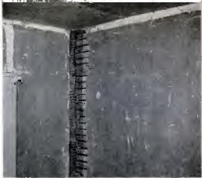
Old plaster has been removed from cracked area at corner of room. Expanded metal lath is nailed in corner and area is replastered along with ceiling
